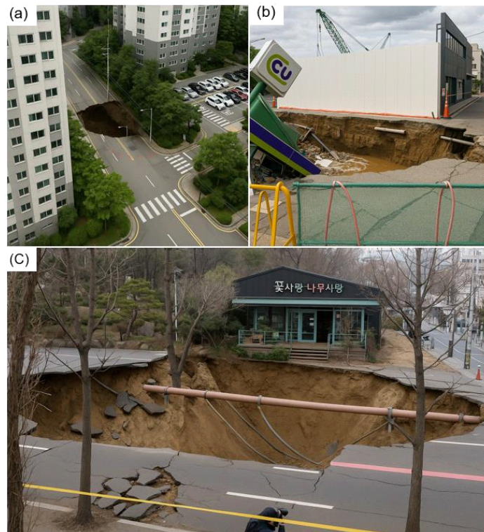
Fig. 5. Recent cases of ground subsidence (sinkholes): (a) Guri City, (b) Yangyang, (c) Myeongil-dong, Seoul. Each image was reconstructed based on photographs reported by the public media; therefore, there are no copyright issues.
