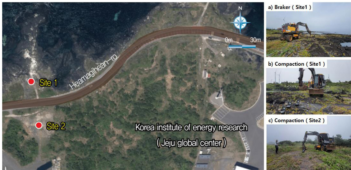
Fig. 2. A location of construction vibration tests and photographs of in-situ tests.
