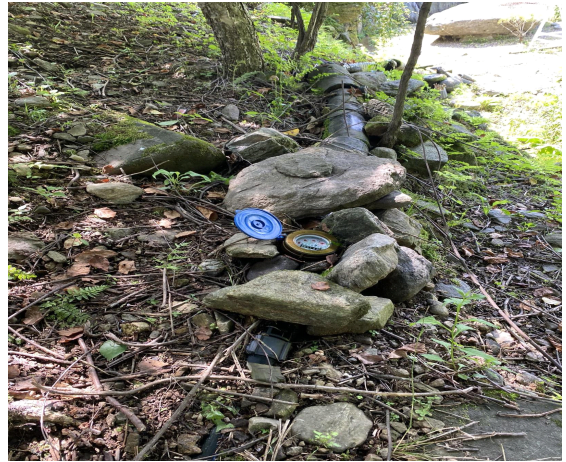
(b) Water tank overflow rate measurement using flow meter
