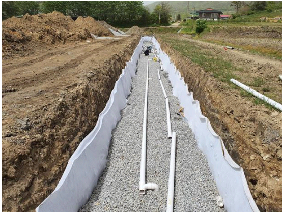
Fig. 3. Combined artificial recharge structure of ditches and vertical wells.
