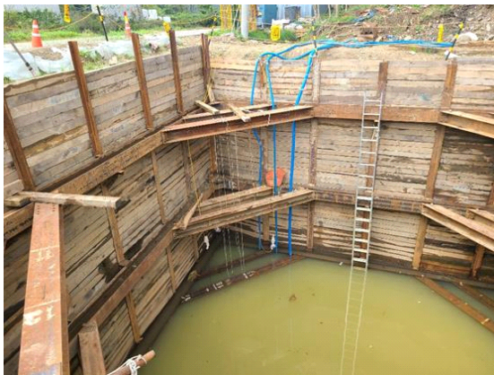
Fig. 4. Combined intake facilities structure of collector well and horizontal pipes.
