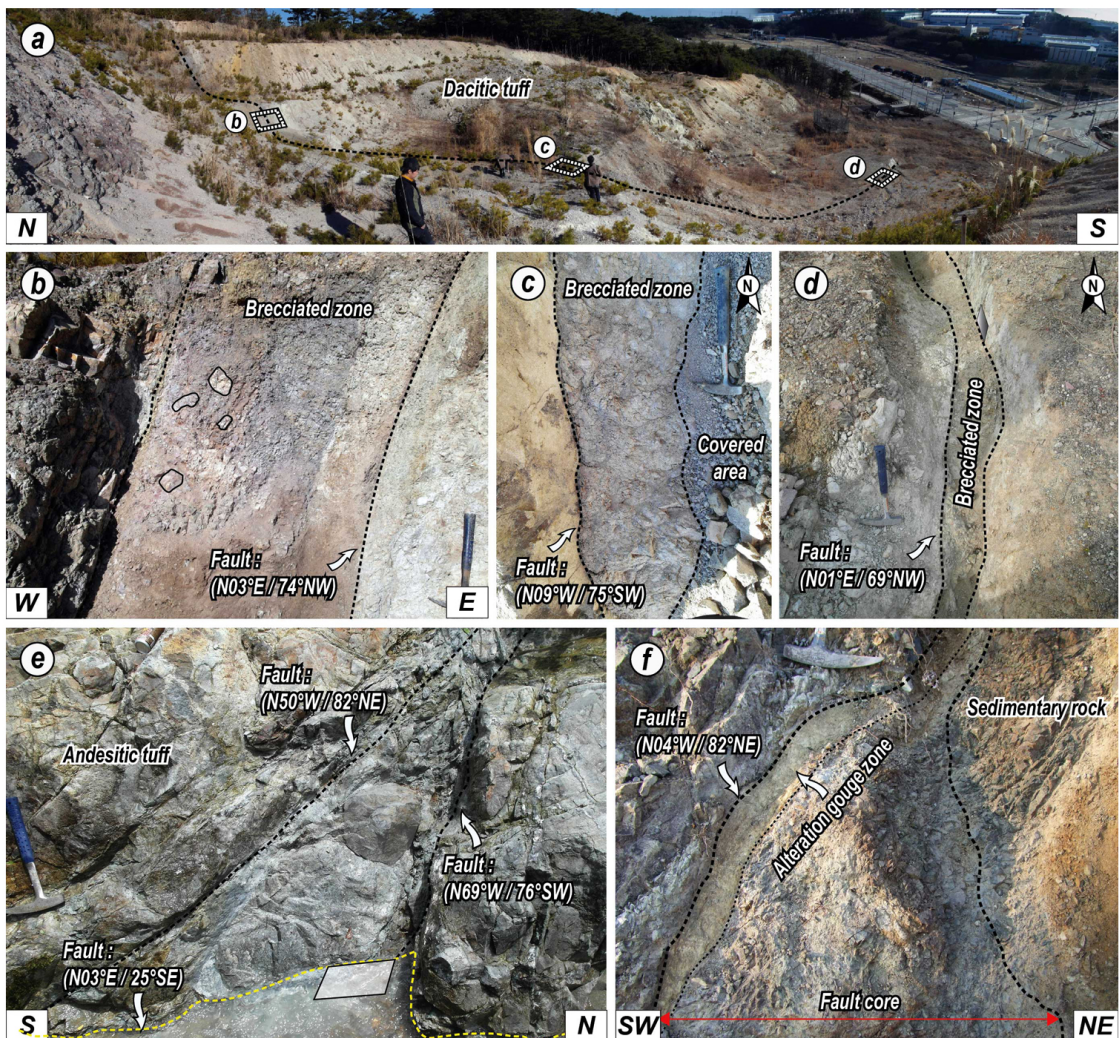
Fig. 9. Outcrop photographs showing major features of N-S-striking faults. (a) An exposure showing about 50 m-extension of N-S-striking fault and (b~d) its fault core composed of breccias, which becomes narrow toward the south. (e) Two WNW-faults offset by a low-angle N-S-striking fault. (f) A N-S-striking fault with ~20 cm-thick fault core consisting of gouge and breccias.
