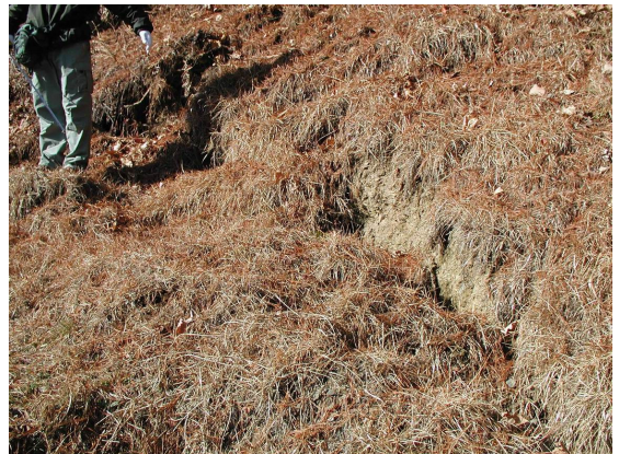
Fig. 5. Tension crack and step in the vicinity of grave.
