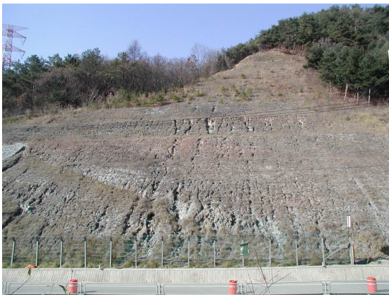
Fig. 6. Surface layer failure at 205 ~ 260 m section.
